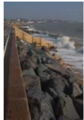
Temporary Sea Defences & beach access
